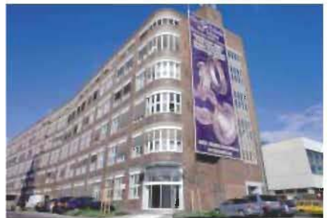
FAG's Aerospace/Super Precision plant in Schweinfurt, Germany
